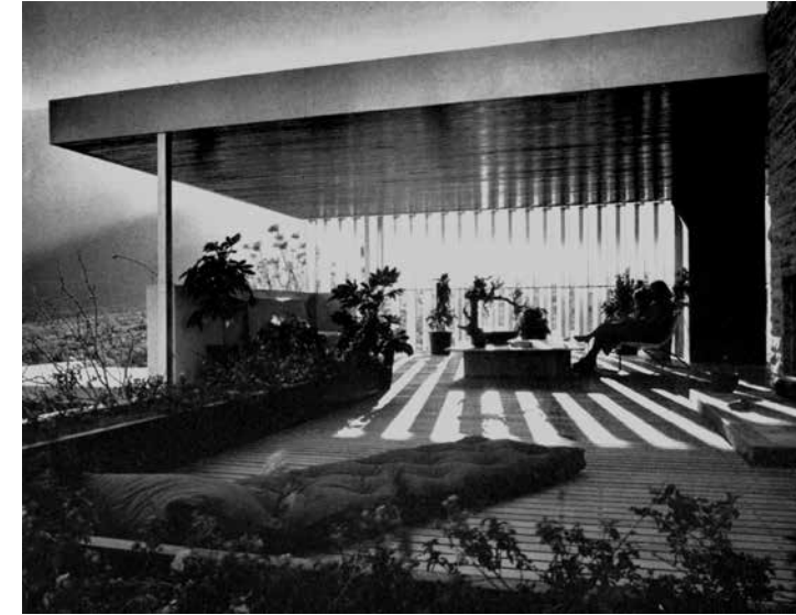
Vertical movable louvers in Richard Neutra’s Kaufmann Desert House, Palm Springs 1946-47 (from: Esther McCoy, Richard Neutra , 1960).
